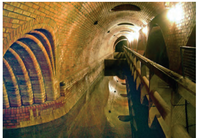
The meticulous brickwork of the settlement tanks and linking passages. Photo Linda Dixon
